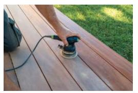
The first step before finishing a deck is to give it a quick sanding with 100 or 120-grit sandpaper. This will get rid of what's called "mill glaze", the everyday marks left on wood by the milling process. This will even out and lighten the colors to prepare them for sealing. This step is often overlooked, but it makes a big difference in the end.
