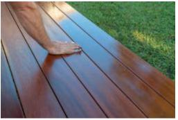
After you finish a section, go back and wipe it dry with a rag. Excess oil will get tacky to the touch if left to dry on its own. If this happens, you can put a little oil on your rag and wipe it up. This will re-wet the tacky area and allow it to be wiped up easily. After you wipe up a section, move on to the next, making sure to overlap the last by a couple inches. It's easiest to work along the length of the deck.
