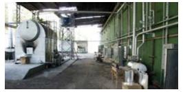
This boiler heats the 12 kilns at our Brazilian facility. We power it using sawdust briquettes and wood scraps to save on natural resources.
